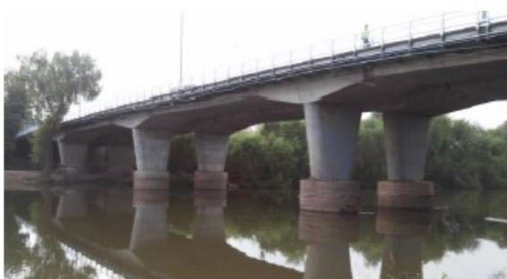
Figure 1. The Juarez Bridge.
